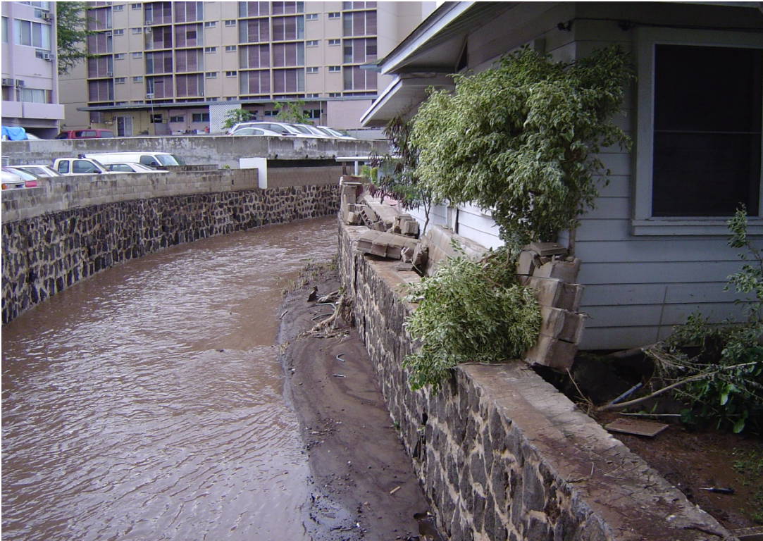
Photo 2. Makiki Stream looking upstream of Fern Street, April 2006 Flood damage to CMU wall built on channel wall from March 31, 2006 storm. Photo by Oceanit.
